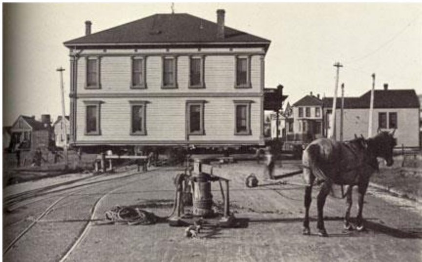
Built in 1884, Berkeley’s first Town Hall was moved in 1899 from University Ave. at Sacramento St. to Grove St. at Allston Way. (Berkeley: The Town & Gown of It)
